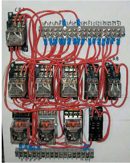
(a) Relay based control panel.(b) PLC-based control panel.
